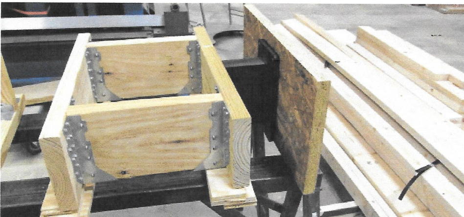
Figure 13: Constructing a Configuration 4 Specimen
